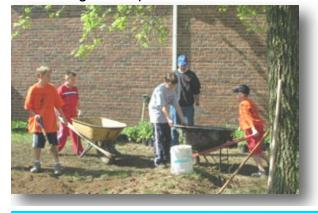
Once the rain garden has been leveled, you can then start adding topsoil and composted organic matter as needed. Refer to page 7 regarding soils and soil composition for more information on soils. Also, shape the berm so that it ties back into the existing landscape and rake the entire rain garden so that it is ready for planting.
