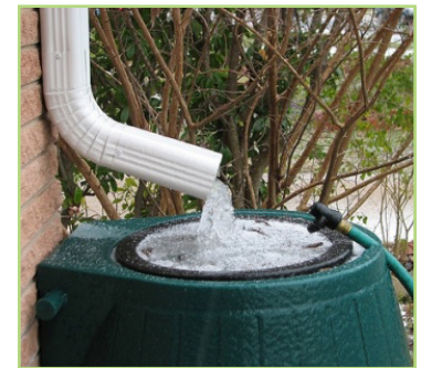
Rain barrels sit conveniently under down spouts to collect rainwater from roofs.
