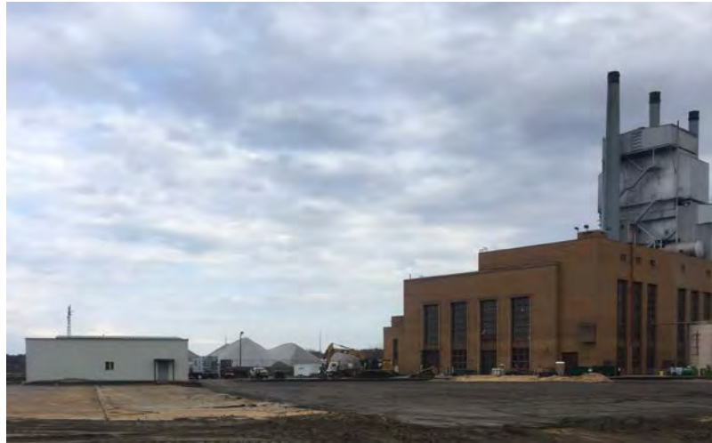
Mid-cleaning of large buried concrete pad
