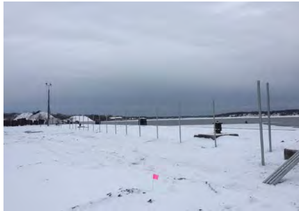
Fence posts along south and west end of property
