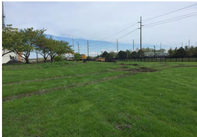
Overview of Test Pits done today
