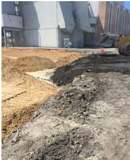
Edge of CCR left in place
