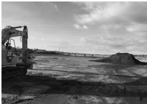
Sand being spread in approved area north of concrete storm structure
