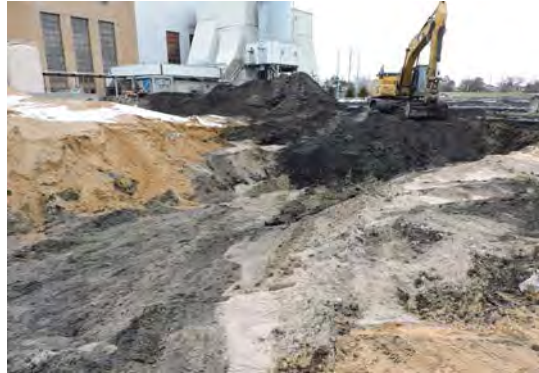
Ongoing excavation of CCR Area just north of Point 4038
