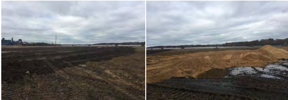
Areas being covered with top soil and sand
