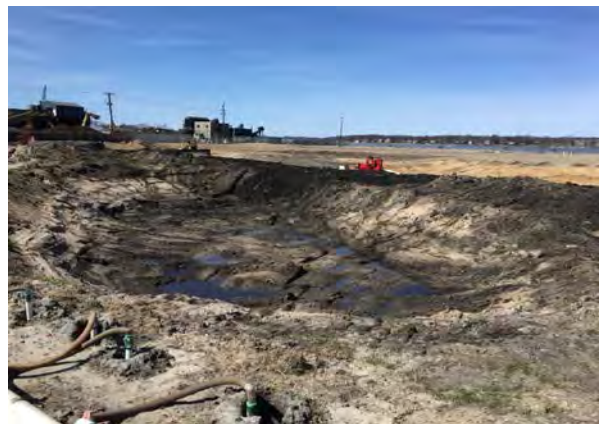
Pond 2 after an additional foot was excavated off the bottom
