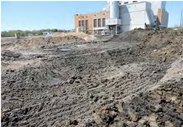
Excavation of CCR material in the newly added CCR area
