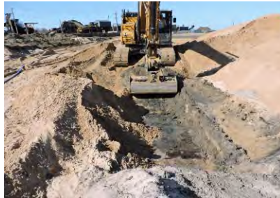
Excavating the CCR material found between Points 4081 and 4082
