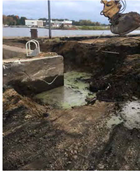
Excavation/Backfill of coal between certification points 134 and 107
