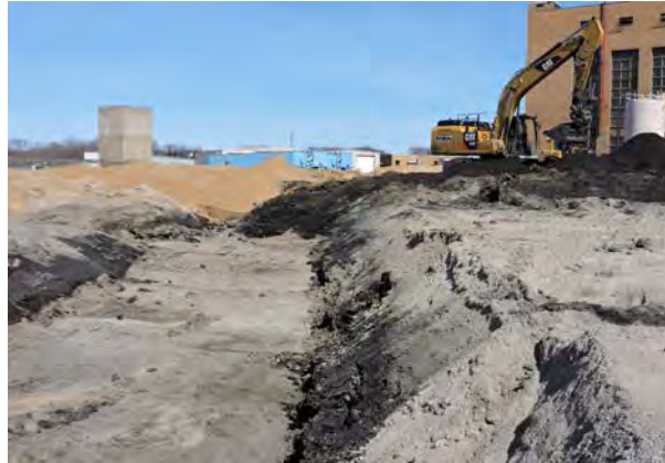
Culvert along Points 4035, 4050, 4051, 4063, and 4073
