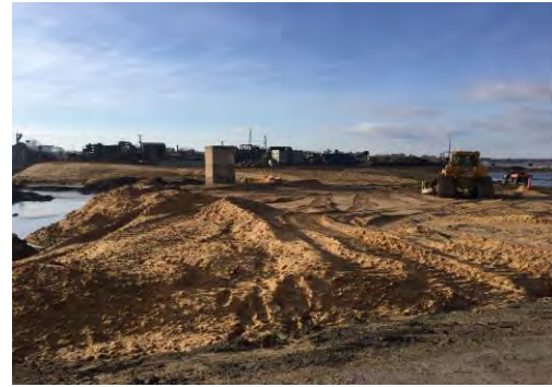
Sand being spread in verified area north of concrete storm structure
