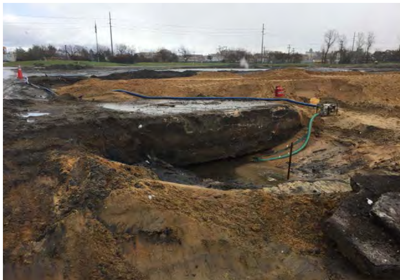
Uncovered concrete pad located between points 4001 and 4002
