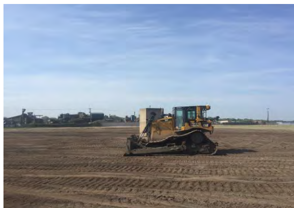
Re-grading of the middle of the site via dozer
