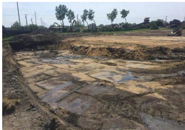
CCR area under excavation
