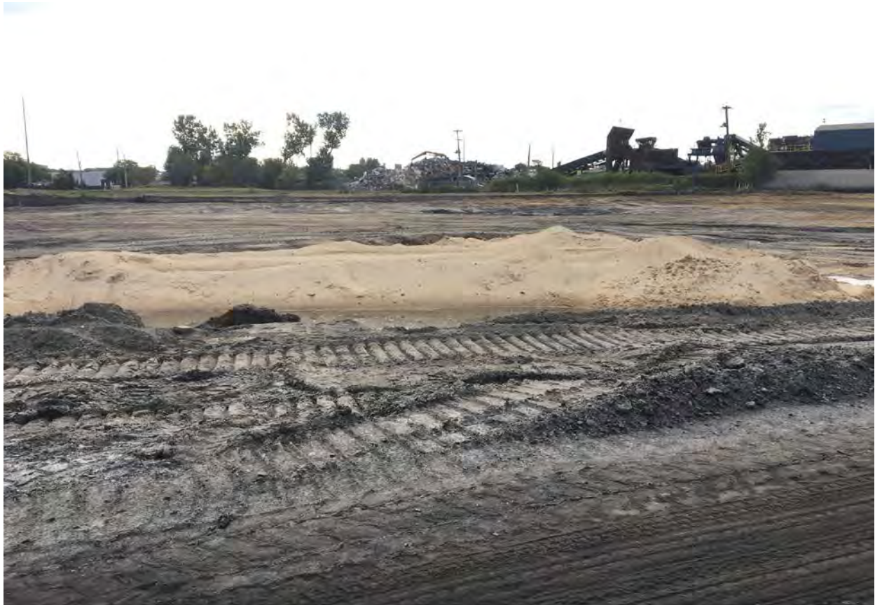
Hopper hole filled with sand
