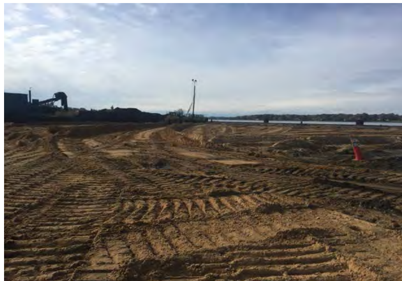
Approved areas being backfilled with sand
