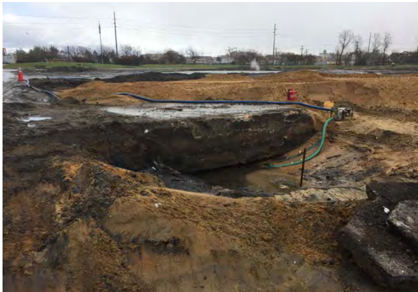
Uncovered concrete pad located between points 4001 and 4002
