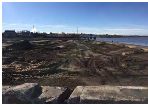
Approved areas being covered with top soil
