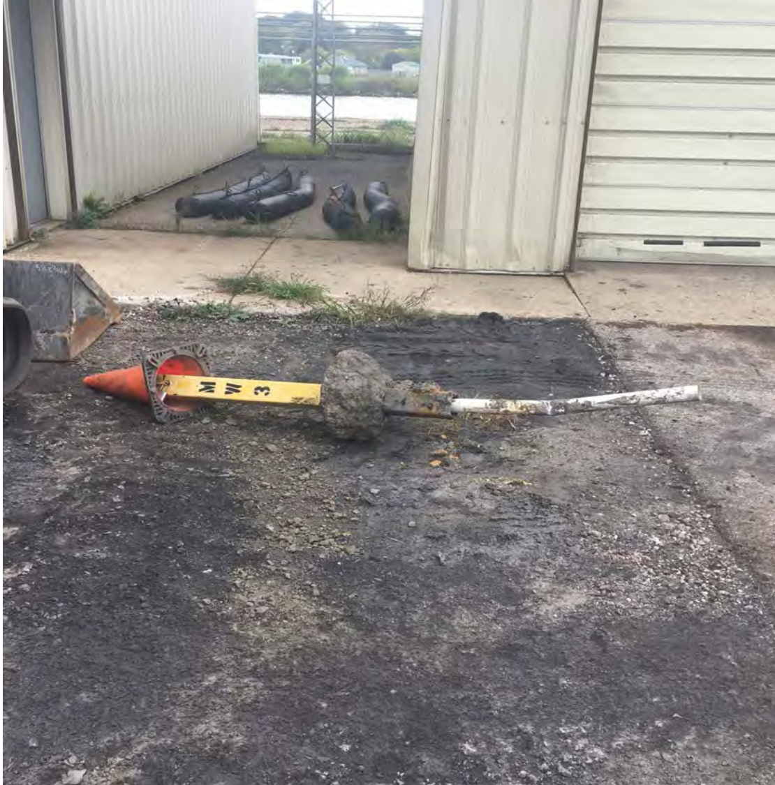
MW-3 after removal
