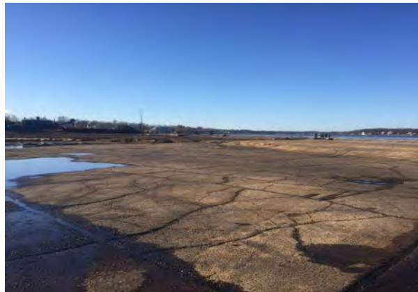
Power washing of large buried concrete pad
