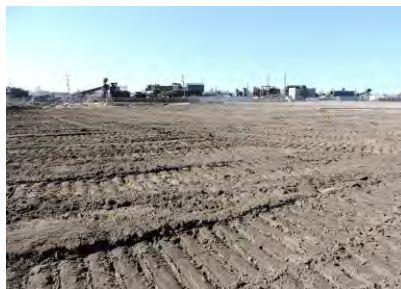
Topsoil along west edge of verified CCR area
