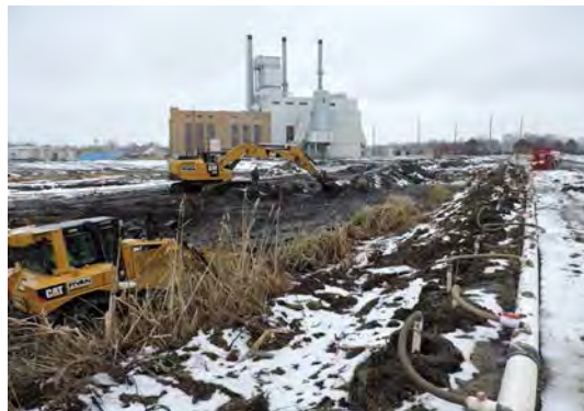
Excavation of Pond 3 CCR Material
