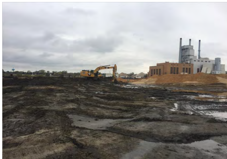
Area being excavated in southwest corner
