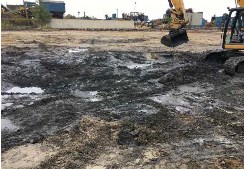
Excavation of slag area in southeast of site
