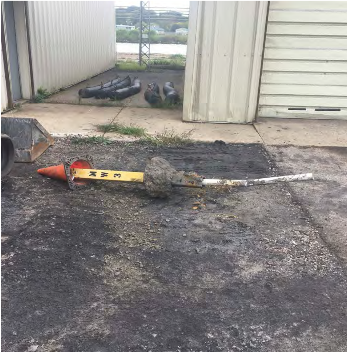
MW-3 after removal
