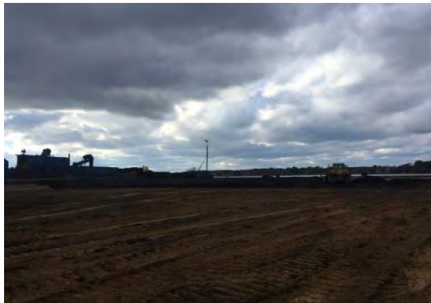
Soil being layered on top of sand
