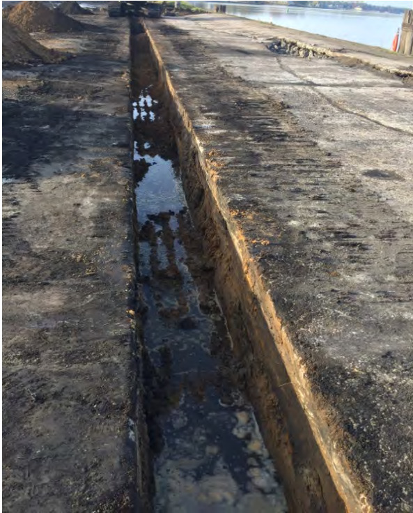
Electrical conduit after removal and during backfill
