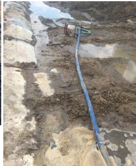
CCR area under excavation
