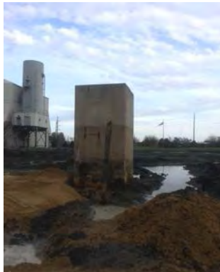
Teeing of leaking storm sewer pipe at the northwest corner of the storm junction box
