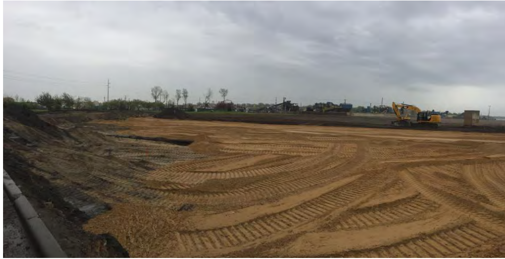
General picture from today's site visit
