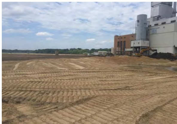
Verified CCR area backfilled with sand
