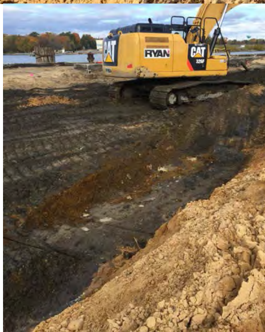
Area between points 4115 and 4110 being excavated
