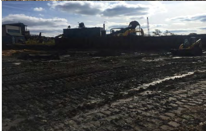
Southwest corner being excavated
