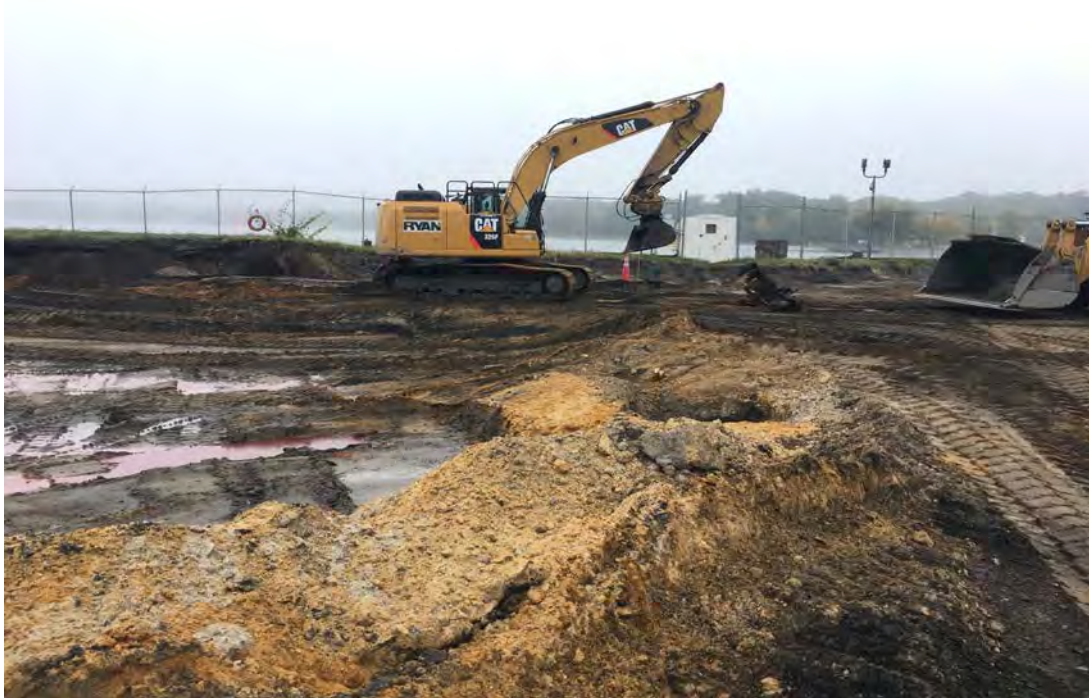
Metal storm pipe being removed on west side of coal yard
