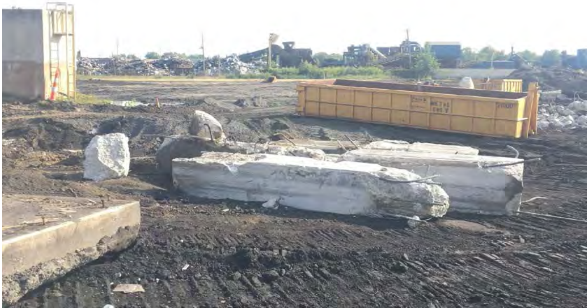
Concrete remaining after conveyor removal
