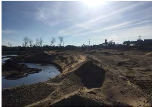
Sand piled along approved edge, to the south of concrete storm structure
