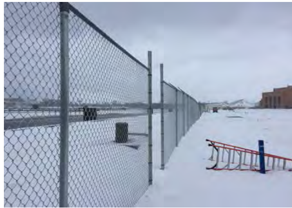
New fence along south and west sides of the property
