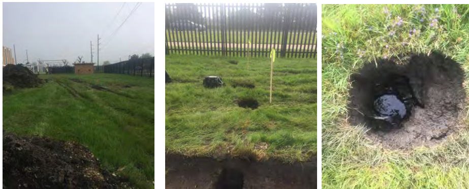
Holes over snowmelt lines
