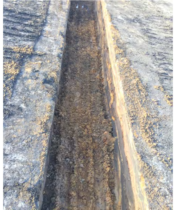
Electrical conduit after removal and during backfill
