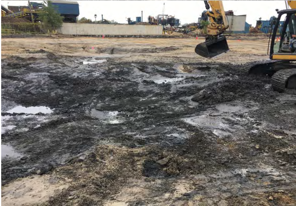
Excavation of area surrounding Point 196
