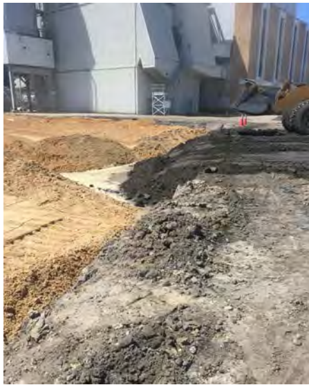
Edge of CCR left in place
