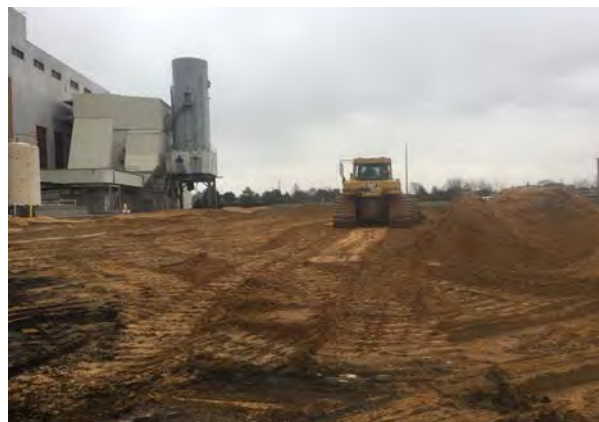
Pictures from today's site visit
