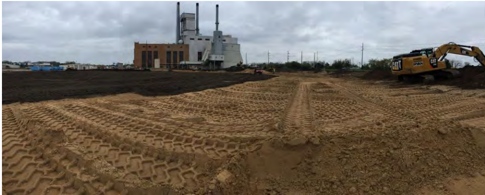
General picture from today's site visit
