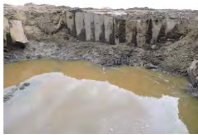
Pictures of excavated weir
