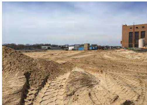
Backfilled area along the northwest portion of the verified CCR area
