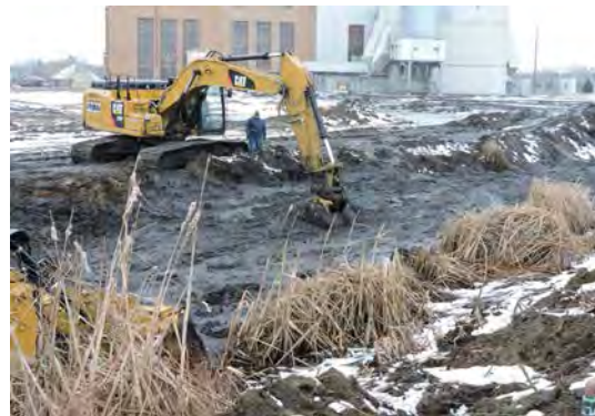
Excavation of Pond 3 CCR Material
