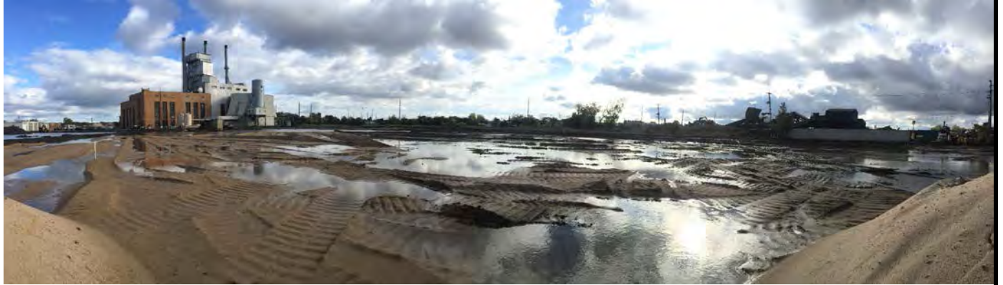
Flooding on site
