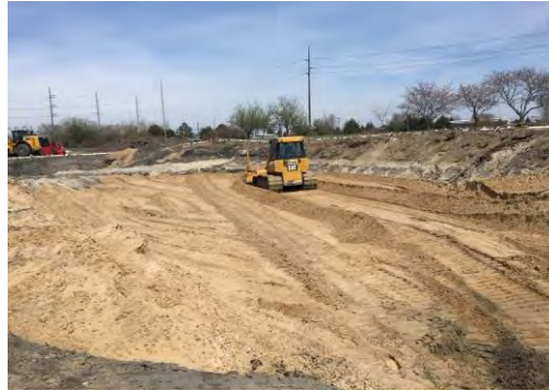
Pond 1 (left) and Pond 2 (right) backfilled with sand
