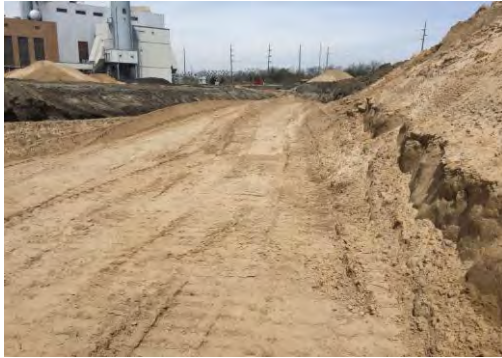
Pond 1 (left) and Pond 2 (right) backfilled with sand
