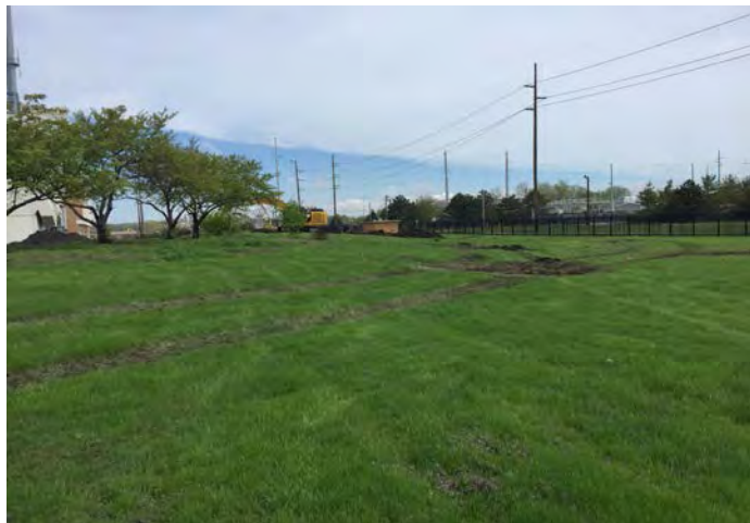
Overview of Test Pits done today
