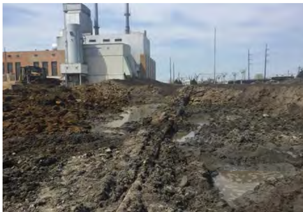
Excavation of CCR material in the newly added CCR area boundaries
