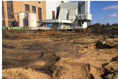
Verified areas being backfilled with sand
