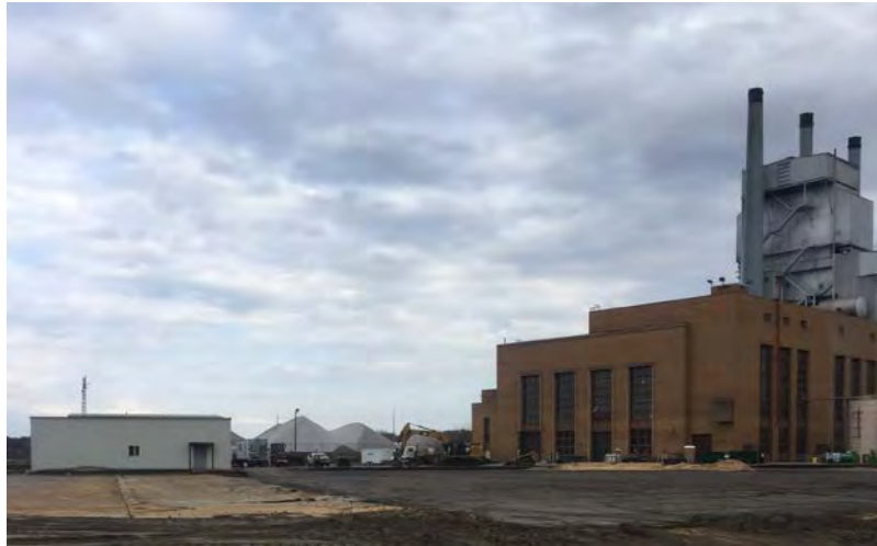
Mid-cleaning of large buried concrete pad
