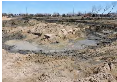
Excavation of area surrounding/north of Point 196
