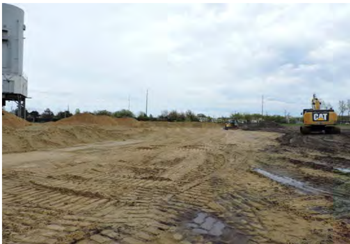
General picture from today's site visit
