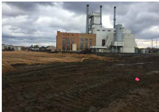
Point 199 / Portion of area excavated with skidsteer
