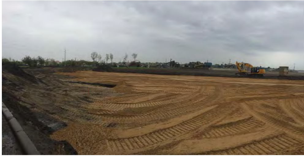
General picture from today's site visit
