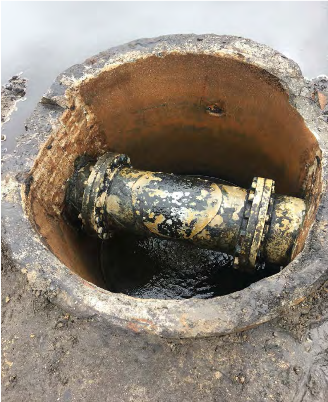
Excavation of manhole by hydro excavators
