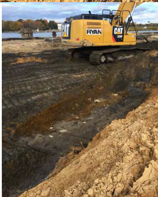
Area between points 4115 and 4110 being excavated
