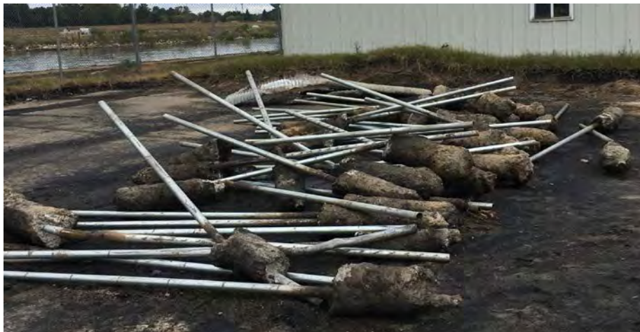
Fence posts after removal
