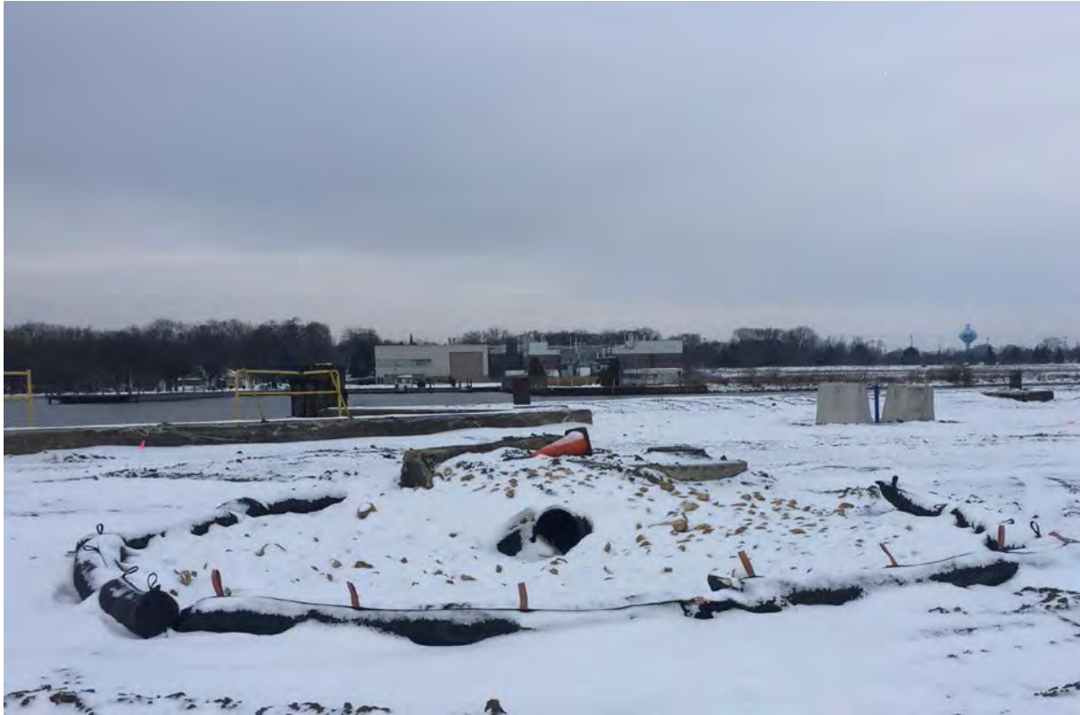
Finished fantail with silt fence
