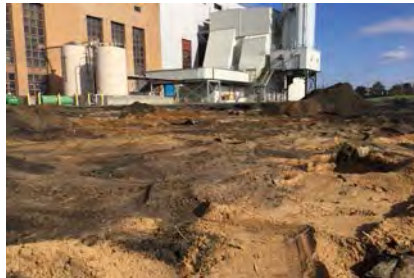
Approved areas being backfilled with sand
