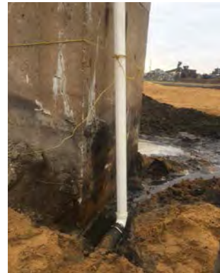
Teeing of leaking storm sewer pipe at the northwest corner of the storm junction box
