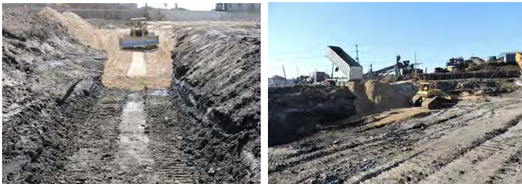
Pond 3 being backfilled with sand
