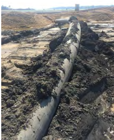
Portion of the dead snowmelt line being demo'd
