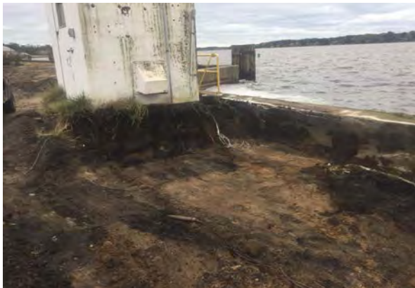
Pump house sitting on a layer of coal
