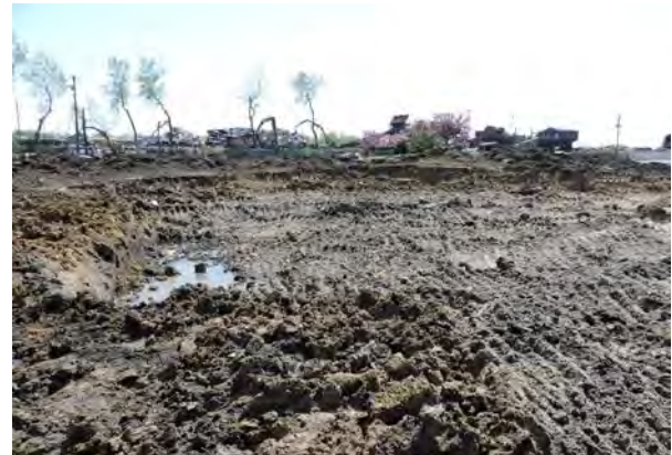
Excavation of CCR material in the newly added CCR area
