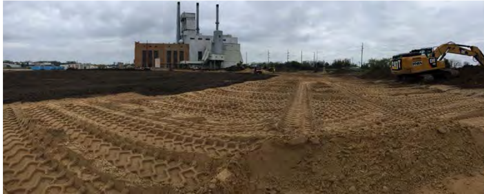
General picture from today's site visit
