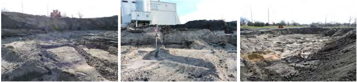
Pictures of excavated bottom of Pond 1 (Have yet to clean walls)
