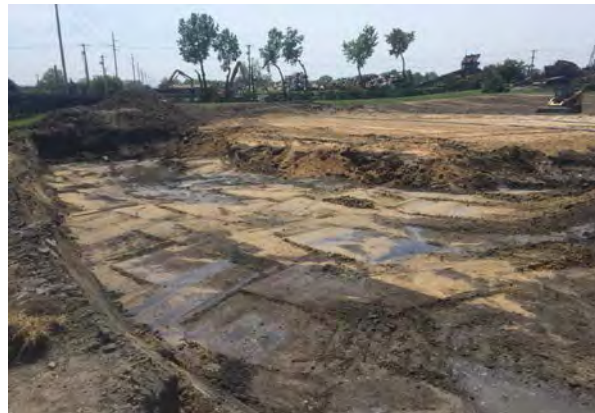
CCR area under excavation
