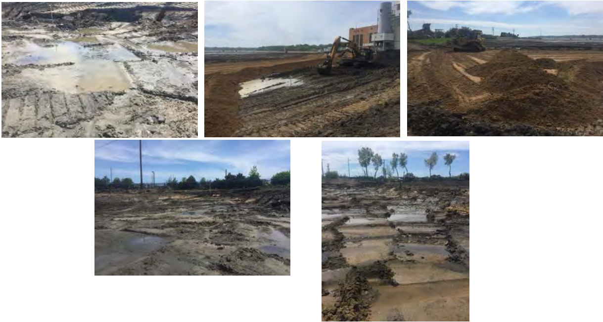
Pictures of CCR area under excavation
