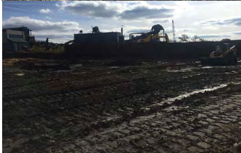
Southwest corner being cleaned
