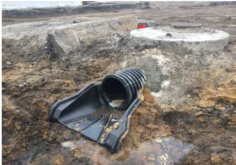
Fantail mid-installation at stormwater manhole (located between points 134 and 135)
