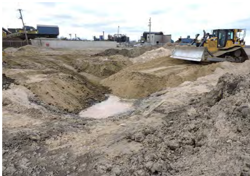
Backfilling of sand near Point 196
