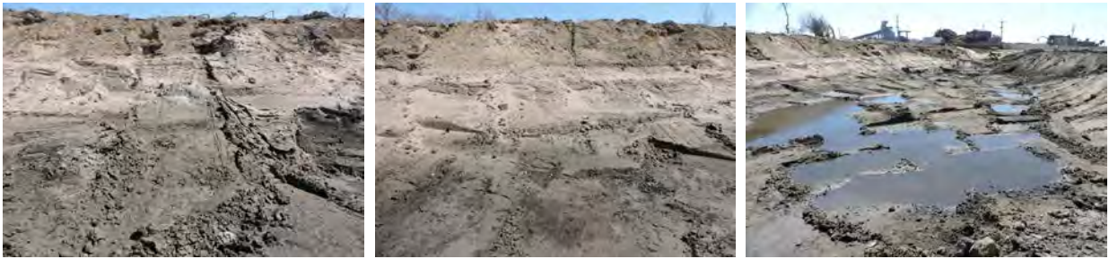
Pond 2 prior to being backfilled with sand
