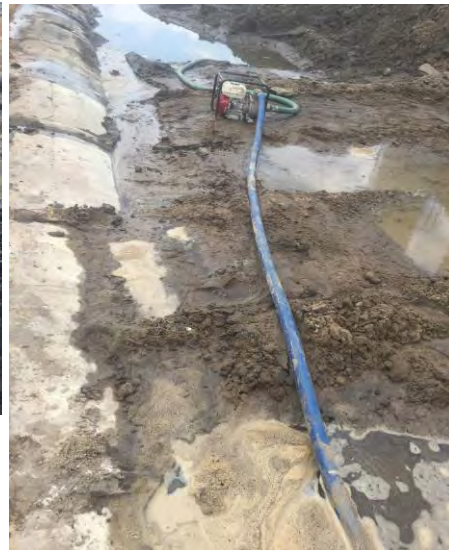
CCR area under excavation
