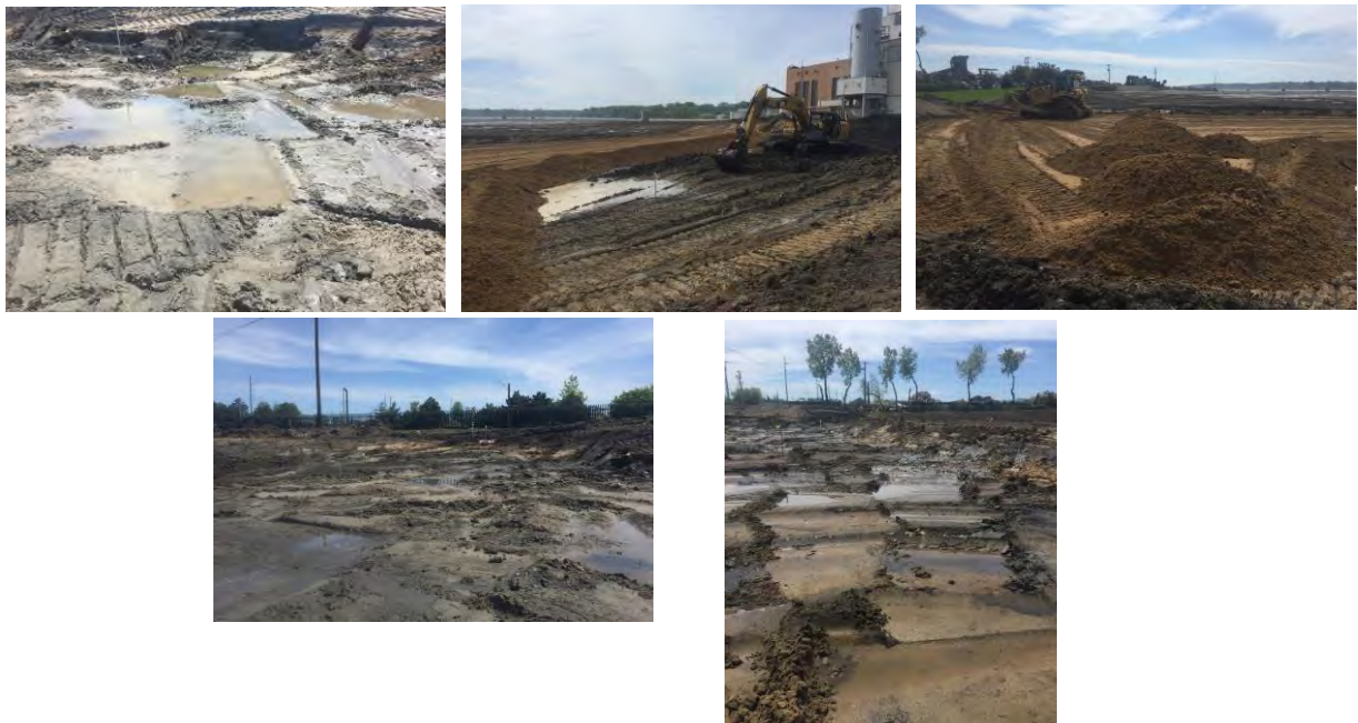
Pictures of CCR area under excavation
