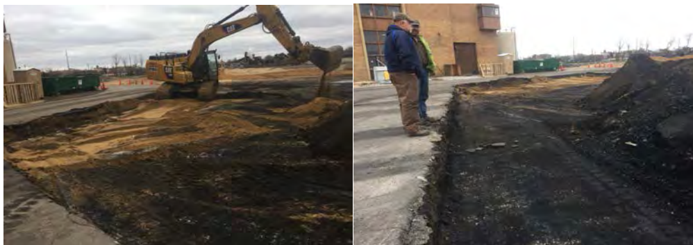
Northern portion of buried concrete being cleaned
