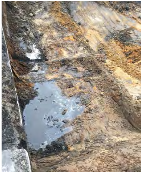
Excavation/Backfill of coal near point 81
