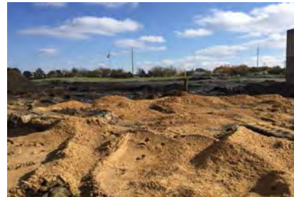
Approved areas being backfilled with sand
