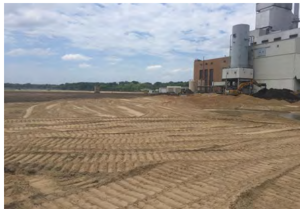
Verified CCR area backfilled with sand
