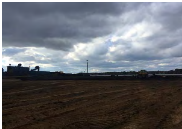
Soil being layered on top of sand
