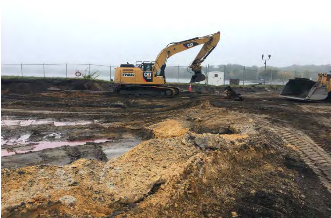
Metal storm pipe being removed on west side of coal yard
